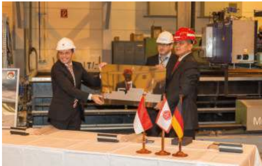
On 26 November 2020, steel for the first mine countermeasures vessel based on the German Navy's Frankenthal class was cut for the Indonesian Navy. (Photo: Abeking & Rasmussen)
